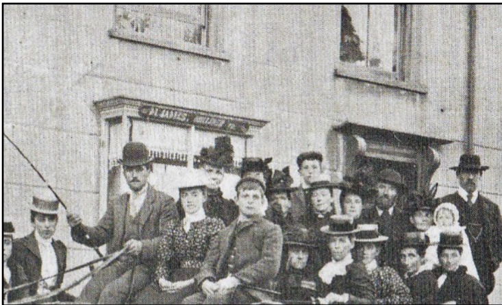
LEFT The upper windows were sash windows, and below is a dainty bay window which was the shop window. A sign there says M JAMES MILLINER. On the top section there is a blind with bobbles partly pulled down (From 'Bro Dafydd ap Gwilym' by David Jenkins, Aberystwyth Public Library)
