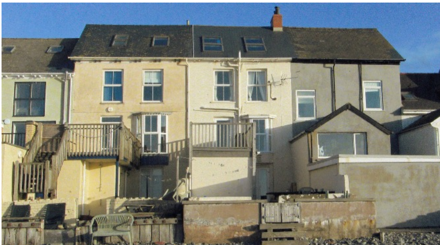
LEFT The rear of Windsor House has the same roof height and placing of windows as Hafod (formerly Ragland) next door on the north, suggesting these two houses may have been built at the same time. The rear roof like the front has an overhang and pairs of dentils. The oriel bay window matches the
