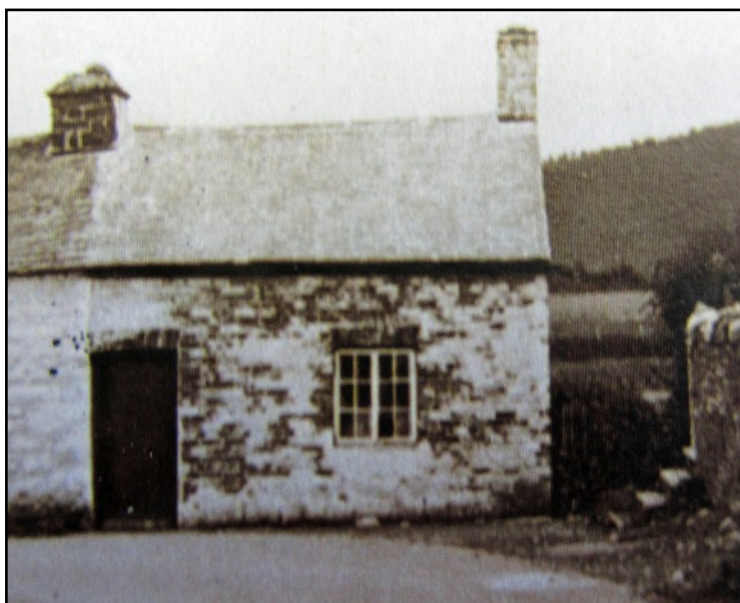
LEFT This photograph taken in 1937 shows the front of her house. The tall brick chimney was for a fireplace with a range for her 'parlour' downstairs at the back. The front door began at the party stone wall.
