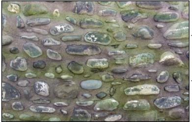
LEFT The rear wall on the north side is rubble stone with a very high proportion of rounded stones from the beach. This kind of wall is found in Borth's oldest cottages. The rubble stone wall ends higher than the front wall of Wesley Cottage. It may have been re-used from an older building.
