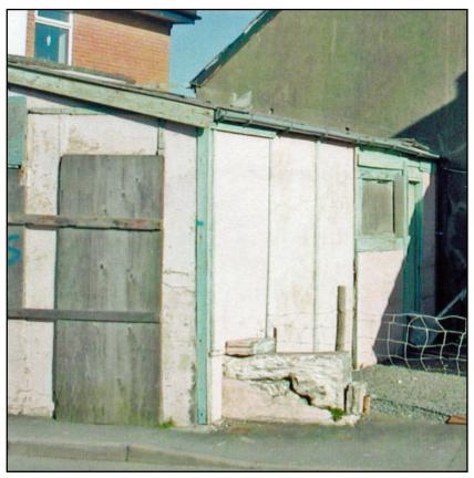
the eaves of the building. The roof is of a very low pitch and covered with corrugated iron - two sheets were needed for the slope. There is access to the building on the south side - between it and Wesley Cottage.
