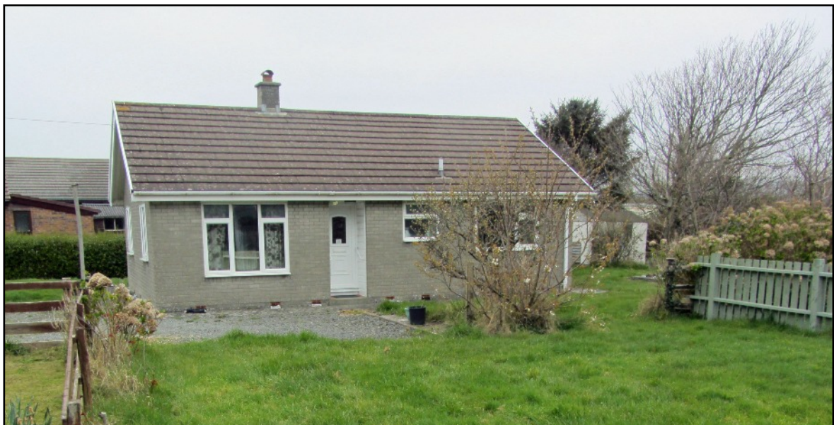
ABOVE The front door of Maes Nant opens on to the open area behind Journeys End and West Wind.
