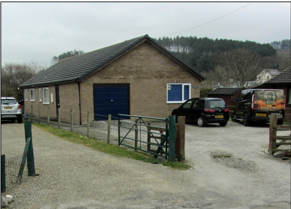
ABOVE Glimar. This has a built in garage.
