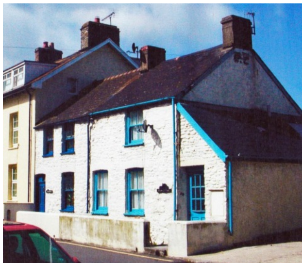
The pair of cottages. The spacing of some of the ground floor windows and the doors suggest they may have been built at the same time.
