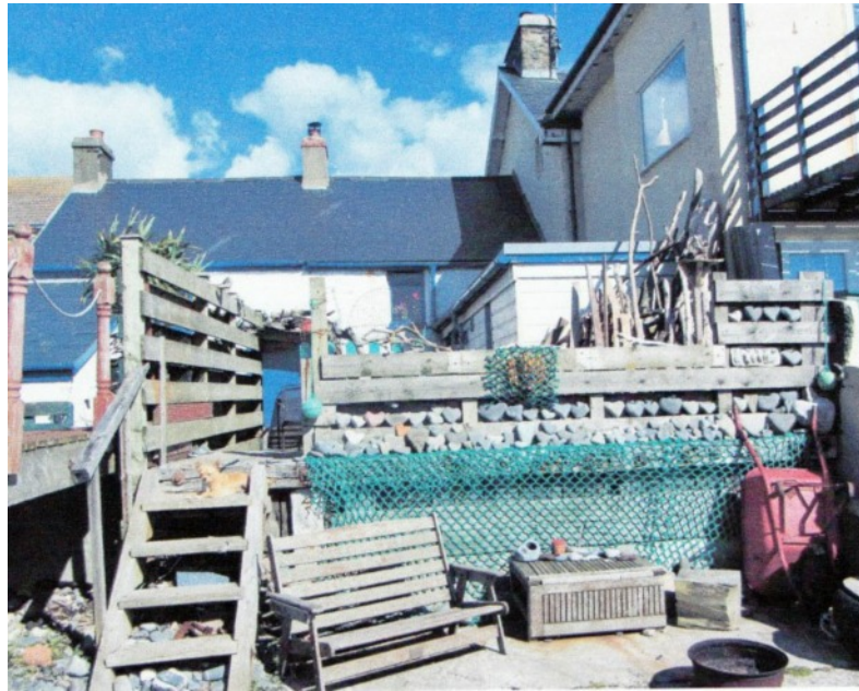
The rear of the cottage from the beach in 2015. The single storey extension with a boarded side and the kitchen and bathroom inside, is on the right. A raised platform for the yard was some protection from the sea during storms.
