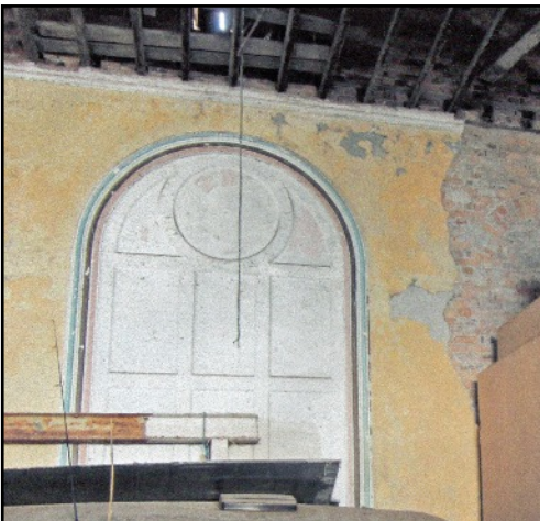
LEFT This window would have been the east window of the chapel, but it is blocked.
