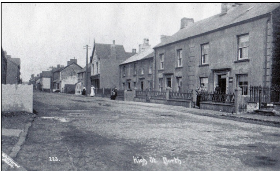
LEFT An early twentieth century postcard by 'Williams of Borth' shows the house with the old sash windows of four lights and with thin glazing bars. In the rendering there was a bold pattern of quoins, and a frame made around each window. The decorative pilasters beside the front
