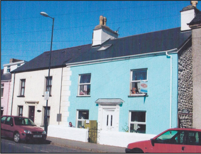
LEFT The house in 2009 showed rounded beach pebbles in the south wall and with two chimneys each with two chimney pots (flues) plenty of rooms could be warmed. The house is very much one of a pair with Beatrice built for a master mariner about 1861.
