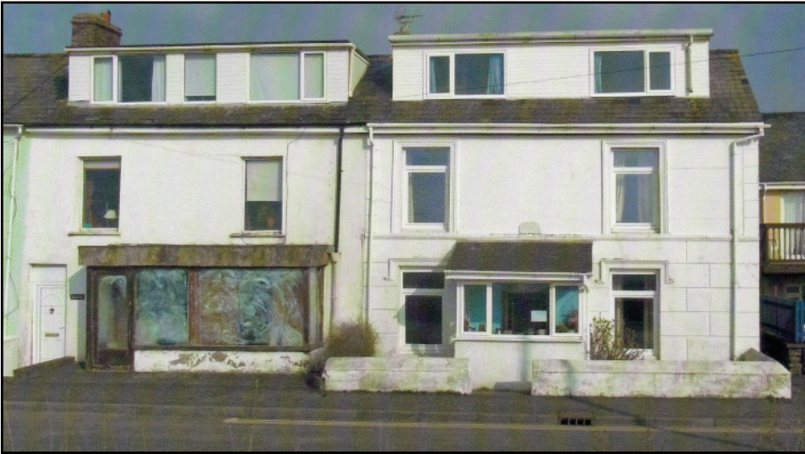
LEFT Efelwen on the right has larger windows with different spacing. Trevayne House opens on to the pavement.
