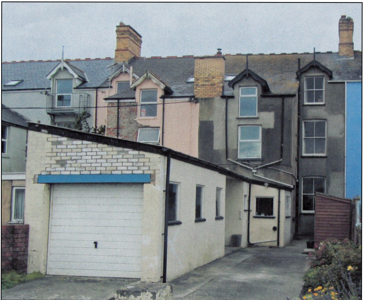
ABOVE The back of the house from the track or lane that runs behind the terrace. The rear is rendered grey. This house like Montfort has an extension on the south side of the back and the main roof extends forward over it. The dormer windows match those at the front of the house. The windows on the extension are modern, and this brick chimney is unique to the terrace, and is shared with Hazelmere. On the roof is one roof light for an attic. There is a line of single storey lean-to buildings in the yard with a roofed central part protecting the back door and ending at a garage. A red brick wall encloses the yard.
