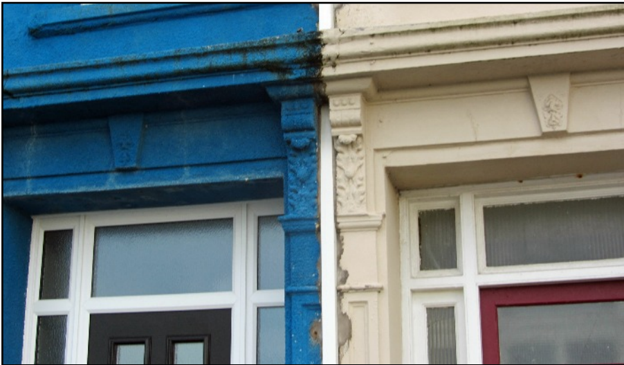
LEFT The brackets supporting the moulded entablature have attractive details, and the keystone too is decorated. These match those of Hazelmere on the right, and Montfort.
