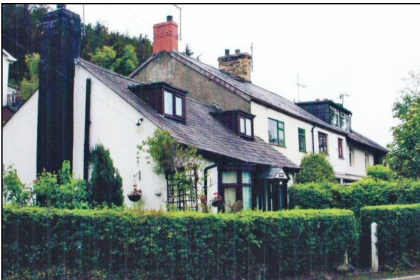
LEFT On this view it is the second tall house along and it has a distinctive yellow brick slab chimney with two chimney pots.
