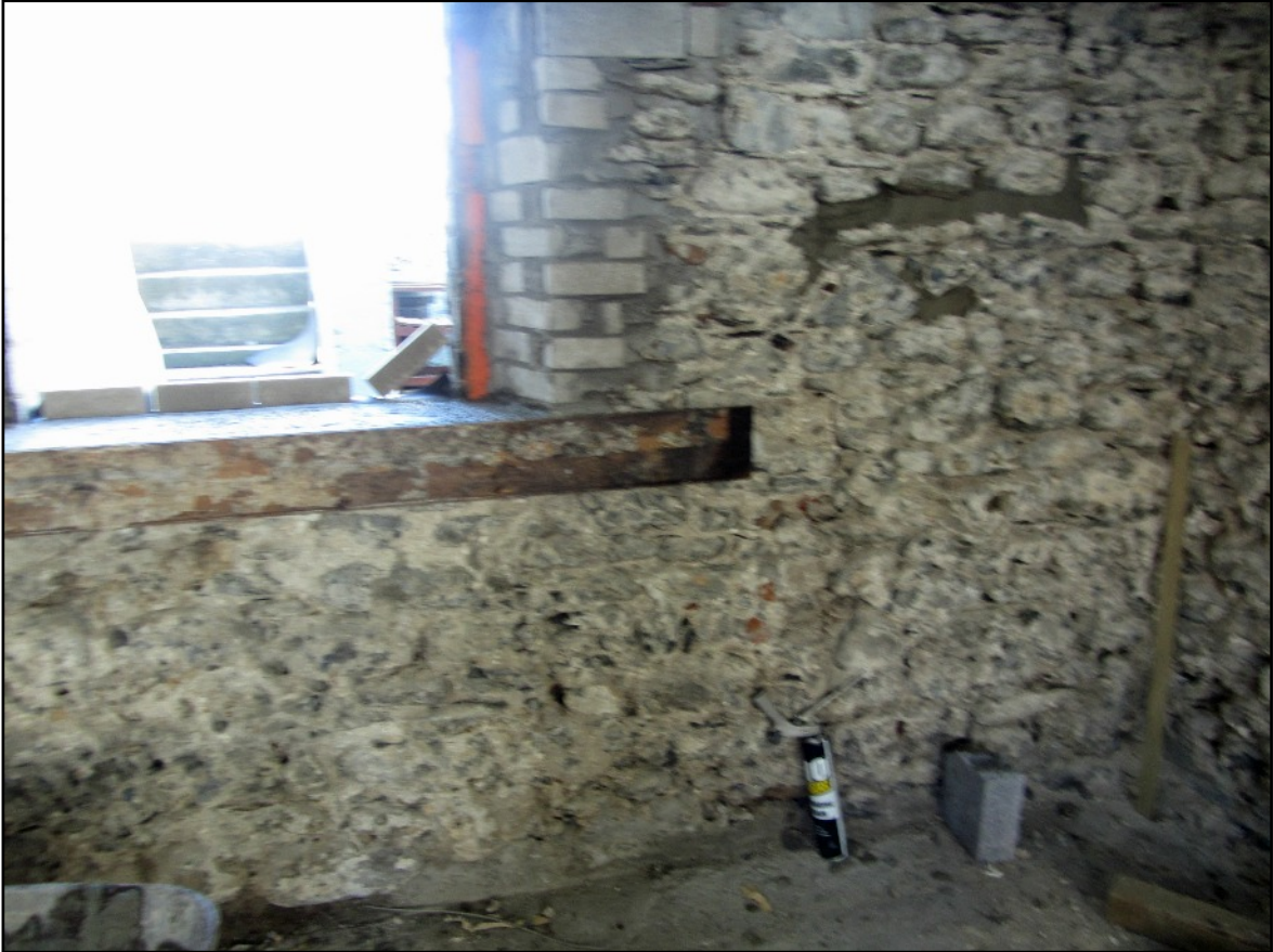
ABOVE This window at the rear of the Art Shop had been edged with bricks and could have been added. Old cottages on the beach side often had a solid back wall to protect them from the sea.
