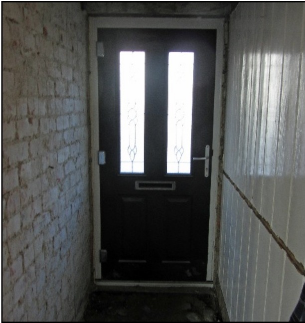
LEFT The front door of Sydney House, and on the left a brick wall had divided it from The Art House next door.
