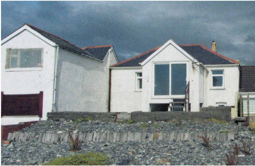
The rear of the house from the beach in 2015.
