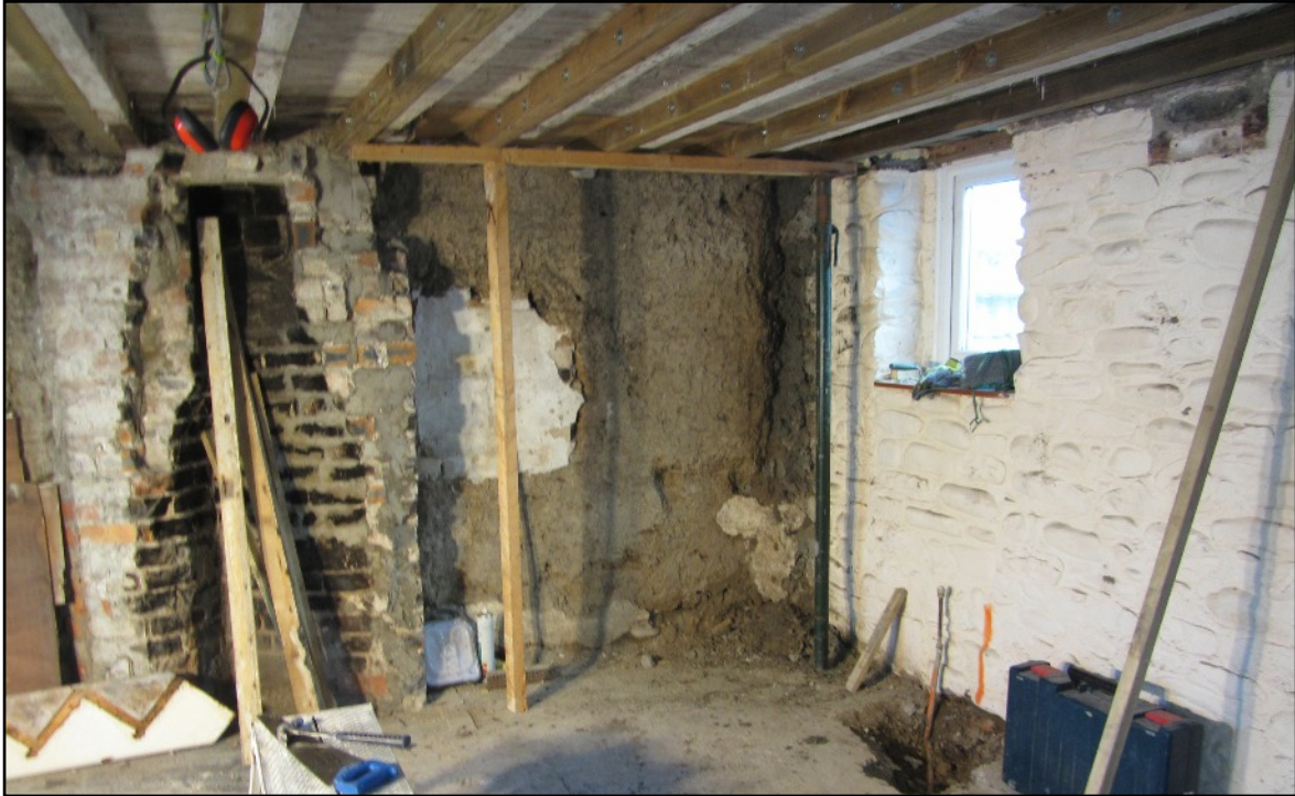
ABOVE A close up of the mud wall in Sydney with just a glimpse of the stones in the base as building work had disturbed the footing. The rear wall of this cottage had rounded stones from the beach. The ceiling is low for a room above.
