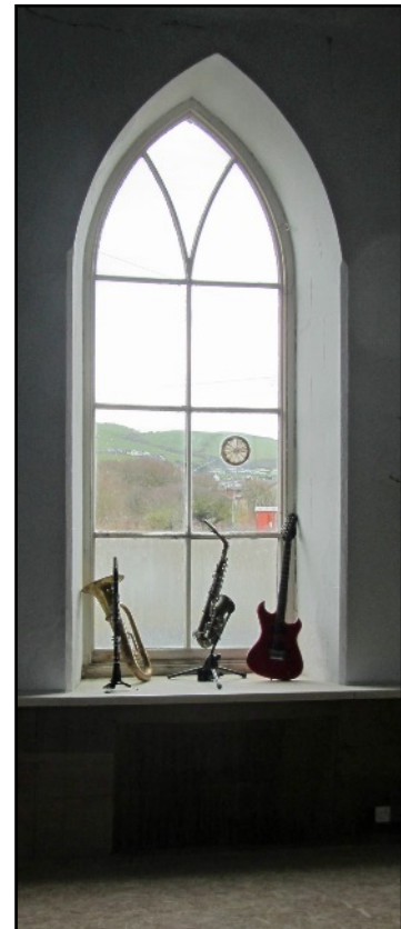
RIGHT The windows have intersecting Y-glazing. There are five each side. This is the window on the south side at the west end.
