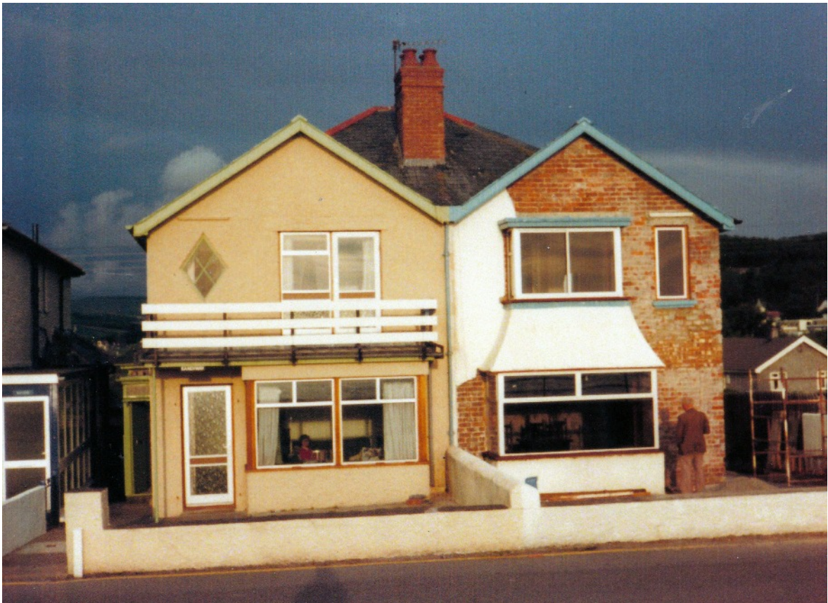
ABOVE This glimpse of the pair of houses shows the bricks which they were built. The diamond shape small window on the upper floor of Sandiway on the left was a bedroom at the time this photograph was taken.
