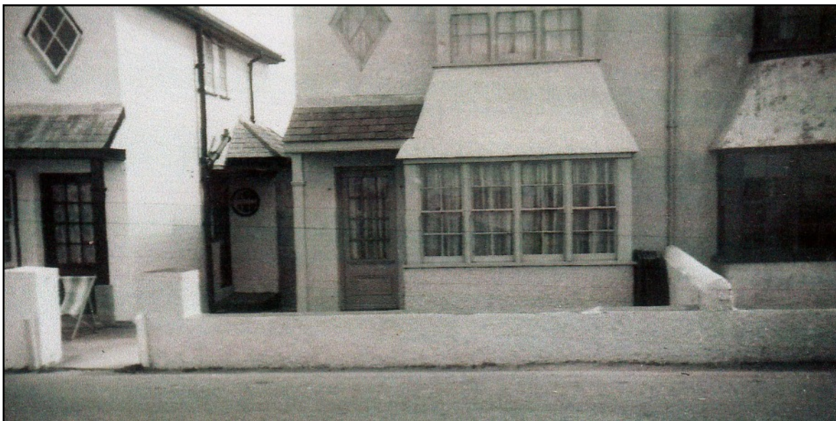
BELOW Lawrence Cash's Sandiway, with possibly its original windows. Today the prominent roof above the lower bay window and the triangular window have gone (Photograph courtesy of Alan Cash)
