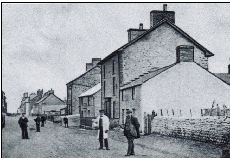
LEFT In the foreground is the cottage in 1906. This is from a postcard, 'Libanus Place'. It had the central doorway and four windows of a cottage, and was one and a half storeys high - the upper windows serving rooms mostly under the roof. The chimney was possibly rubble stone and there were sash windows.
