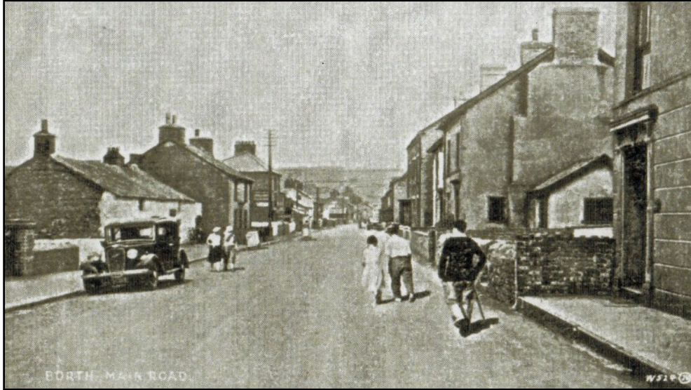
ABOVE This postcard dated 1936 shows from the right the front door of Ynyswen then Beach Grove, and a walled piece of land alongside and then Richmond which already had its porch and front door at the side but no dormer window.
