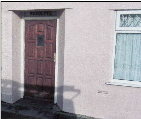
LEFT There is a modern front door and overall a very satisfactory compromise between a 'modern' front and the mock quoins pattern in the rendering which can be seen in the photograph above.
