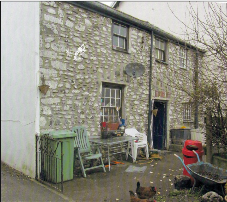
LEFT The rear of the house in February 2015. Some large stones support the outer wall on the left. The back door is wooden and looks old. The door and passage are not central and the spacing of the windows leaves larger rooms on the south side. Some alterations have been made for the top of the left hand ground floor window and over the front door which has a very square top edged by bricks.
