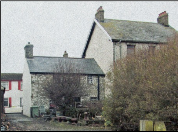
LEFT Pomona House butts against the tall Britannia. Access to the rear is on the south, between Pomona House and Eltham.
