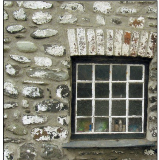
LEFT Inside the right hand ground floor window now of a cloakroom, showing the bricks above the window frame and an arch supporting the upper wall.
