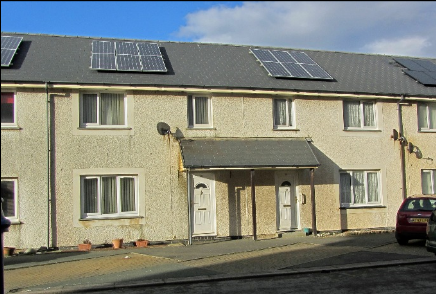
Pantyfedwen Terrace in March 2016. The row leads down nearly to Borth Railway Station, a contrast in red brick.
