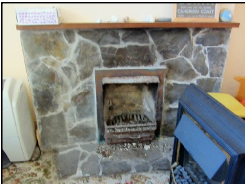
LEFT One fire place on the ground floor is still open. However the surround may not be old.
