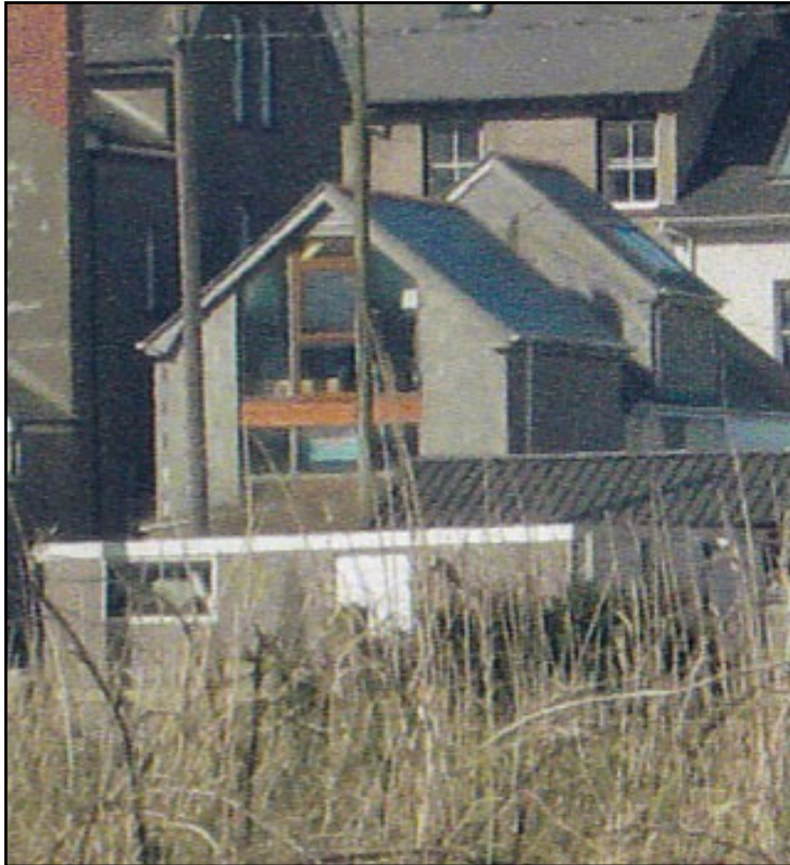
LEFT The rear of the building showing the extension to the roof with roof lights. There are two floors at the back, the upper floor ending with a picture window for the cafe area. This section too had previously been heightened allowing for a spacious workshop below down some steps from the lower floor cafe.
