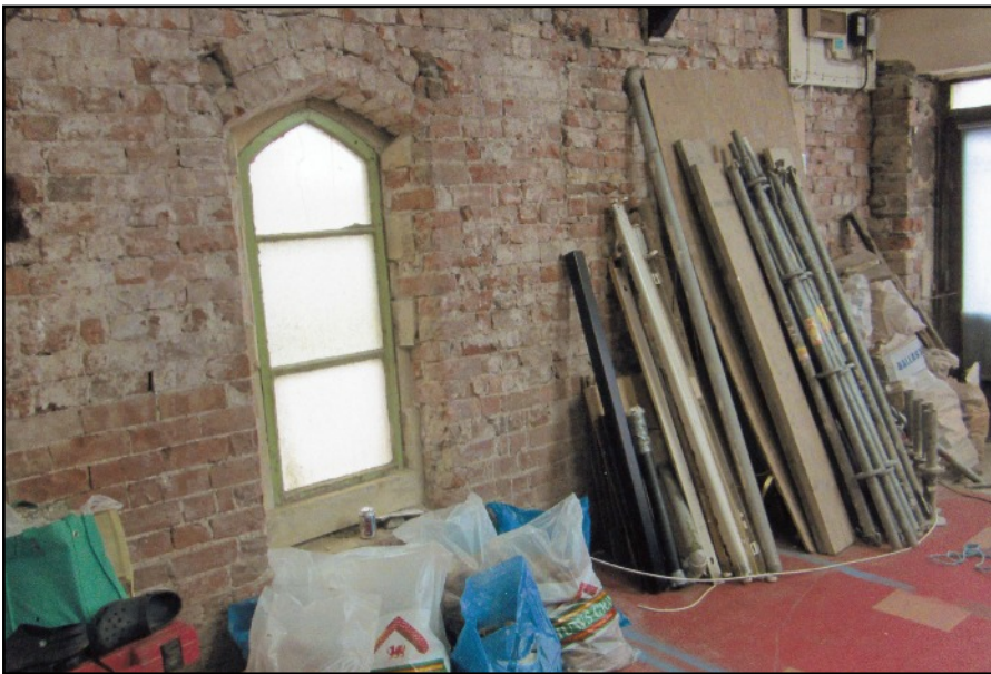
LEFT The inside of the south wall above
