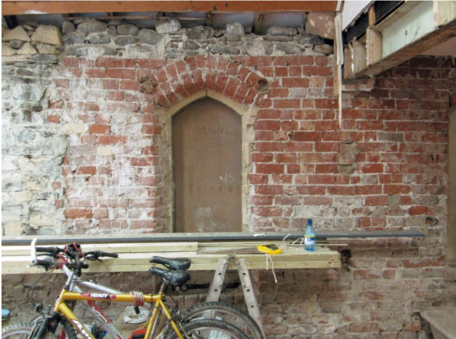
LEFT The window in the north wall encased in bricks.
