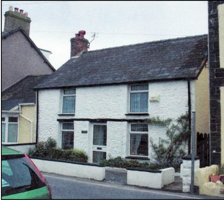
The front of Y Nyth in 2009 and below the rear in 2015.
