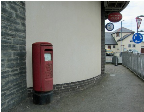
ABOVE RIGHT The footing of the rendered sections of the building is dark brick.
