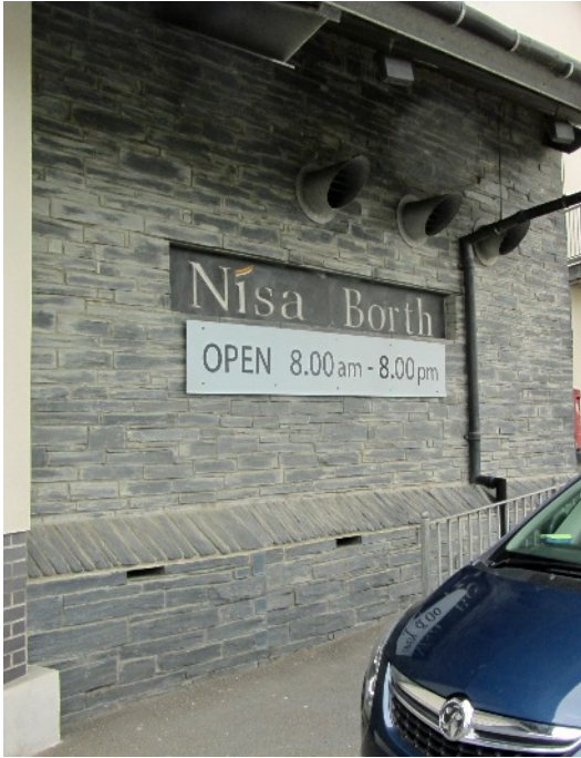
ABOVE LEFT A detail of the slate work and nameplate in 2016. At the very top of the photograph is the end of one of the metal girders used to support the overhanging roof.
