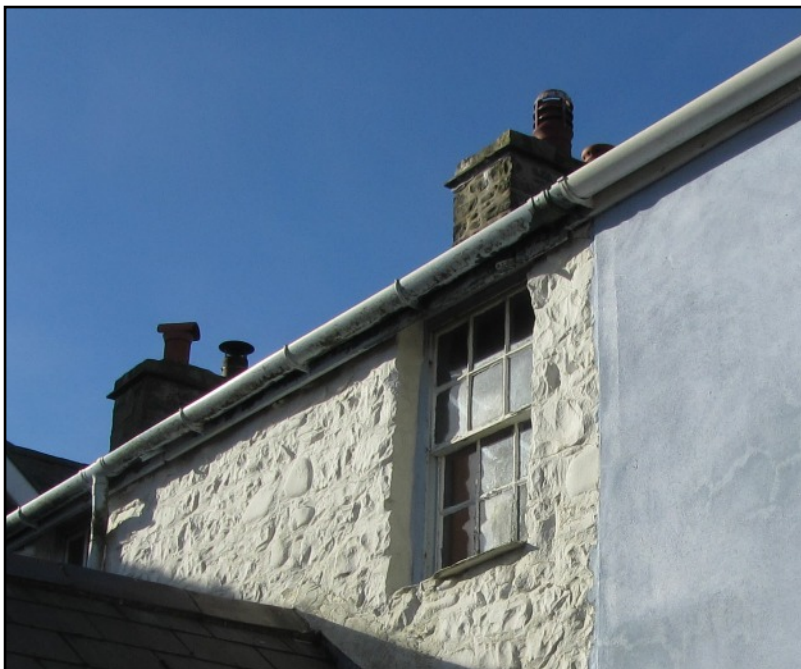
LEFT This is the rear wall of Morfan and shows the rubble stone walling with rounded beach stones - it is likely that all the three houses have walls like this.
