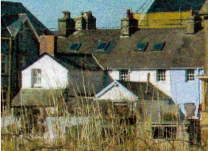
LEFT The rear of the cottages in 2013. Angorfa on the left, and Morfan in the centre, have an attic floor with roof lights. Both have extensions on the rear of the house, Angorfa's is two storey with a brick chimney plus a further lean-to building below. Morfan's is single storey.
