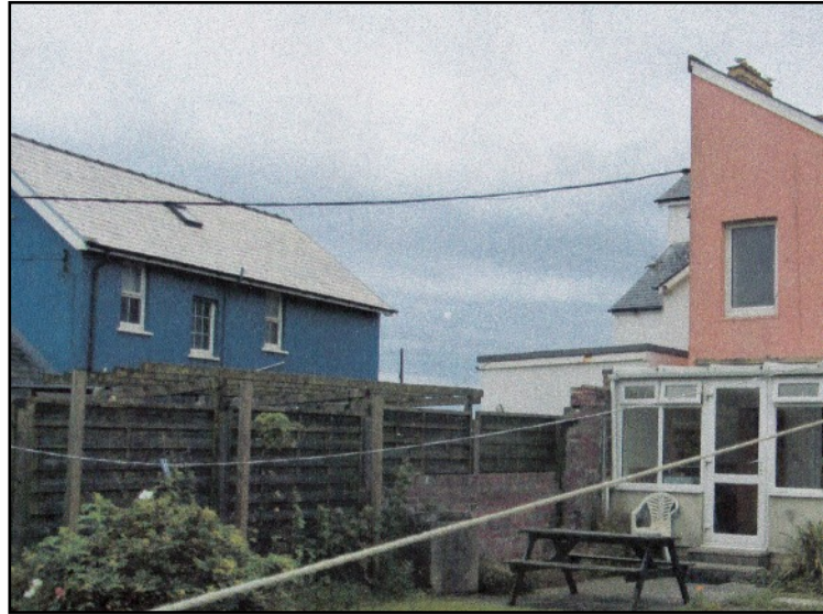
LEFT There is a pattern of bold quoins on the edge of the front wall, and the shape of the string courses is easy to see. This house has no decoration round its windows.
