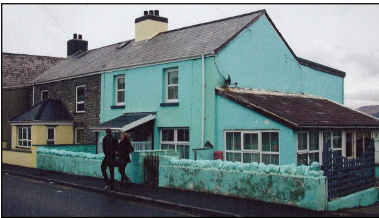
LEFT If compared with The Limit next door the upper windows are set lower, suggesting it may not have been built at the same time.
