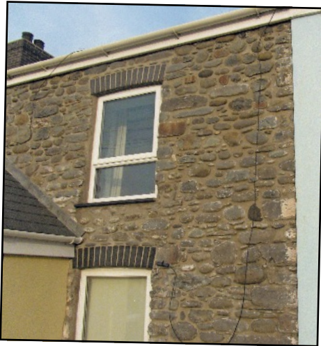
LEFT Some of the rubble stonework is quite random
