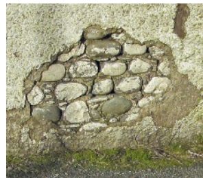
LEFT In 2010 the plaster was being removed on the south wall and there were many rounded beach stones in this wall as in old Borth cottages.
