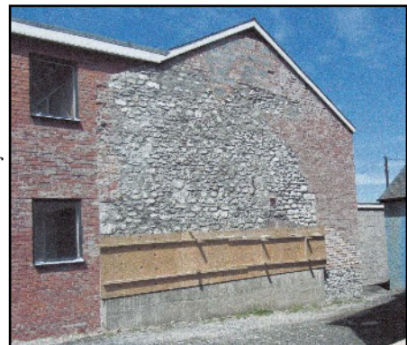
LEFT In 2010 the plaster was being removed on the south wall and there were many rounded beach stones in this wall as in old Borth cottages.
