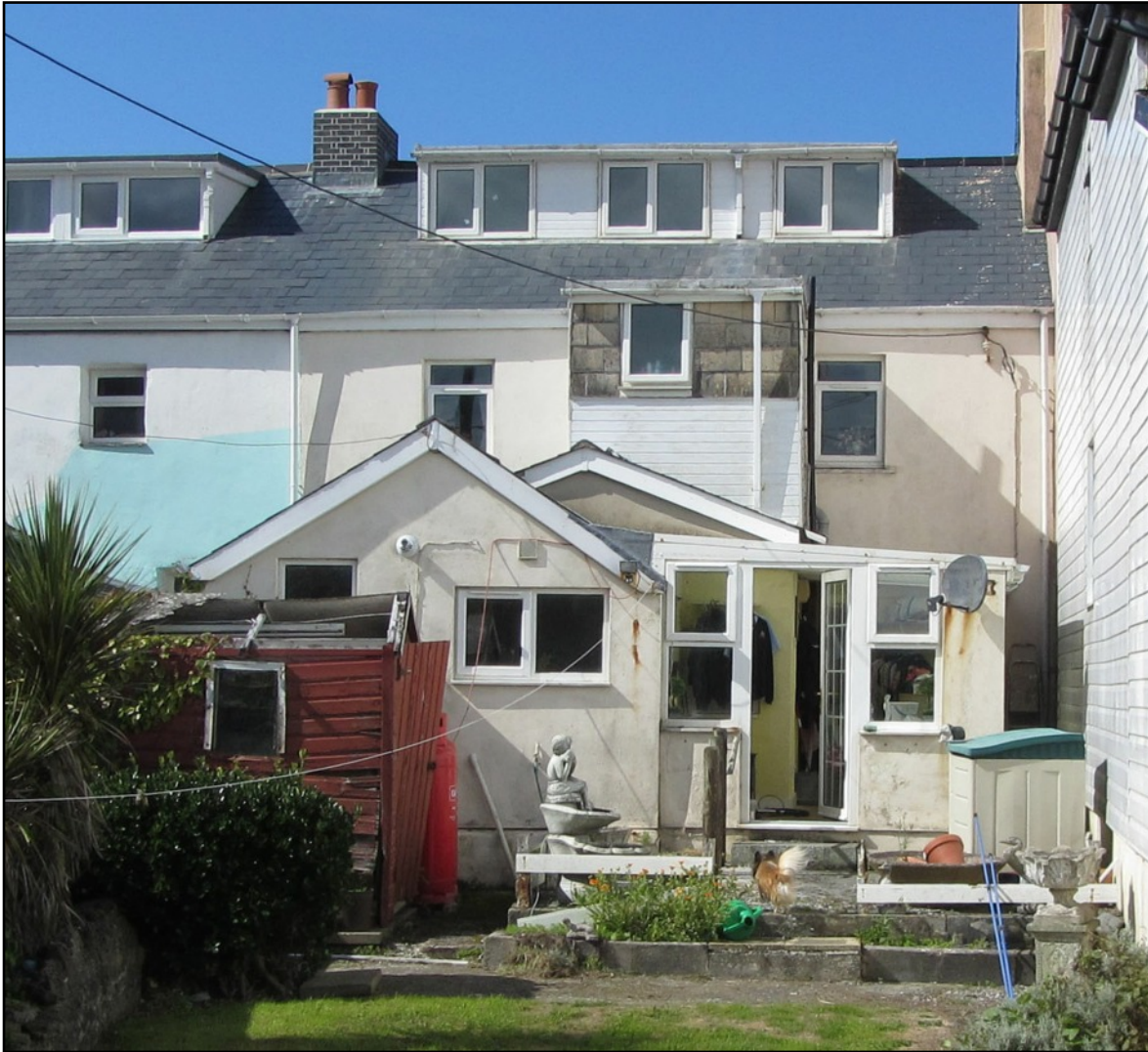
ABOVE The back of the house. Extensions at the back were not there in 1886, but had been built by 1904. They included a kitchen and a Ty Bach inside. The north wall of the extensions butts against Gloucester Cottage. Today there is a glazed porch as well.
