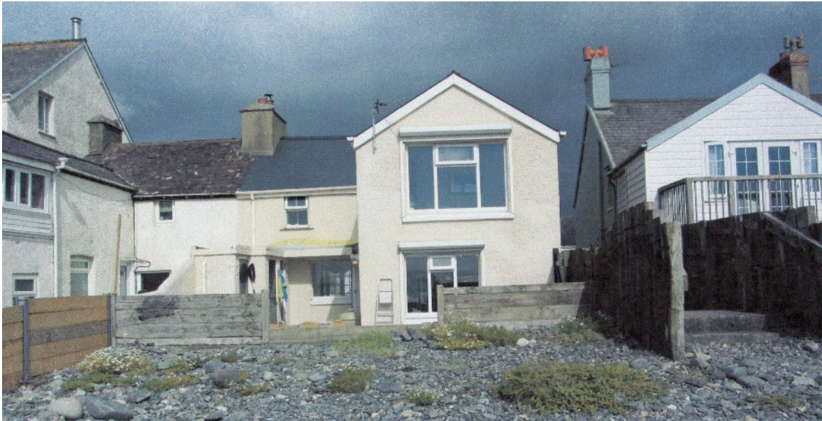
The rear of the house from the beach in 2015.
