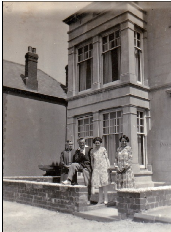
ABOVE This photograph of some of the Herbert family outside Gwynt-y-mor in the 1930s or 1940s shows the south side of Miramar which then had a chimney. There is a glimpse of another chimney.
