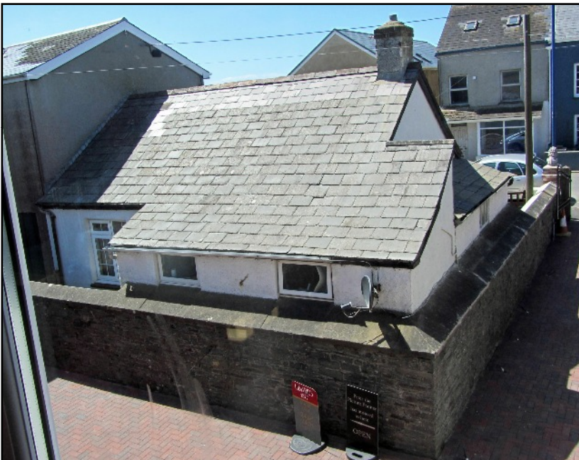
LEFT The rear of the cottage in 2017. There is a roofed extension at the side and the back. In 1886 after the Chapel was built there was only a narrow area at the side and back and the extension partly fills it. The cottage has a right of way into the long garden behind the Craft Cabin.
