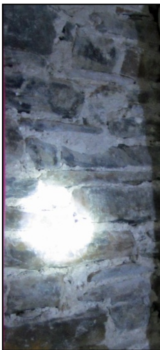
LEFT The walls of this house have quite large pieces of rubble stone in a random fashion. This walling has been exposed on the inside of the front of the house.
