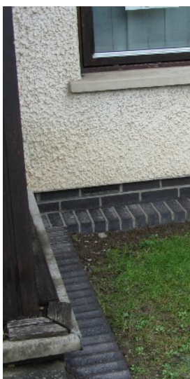
ABOVE The footing of the building is dark bricks.
