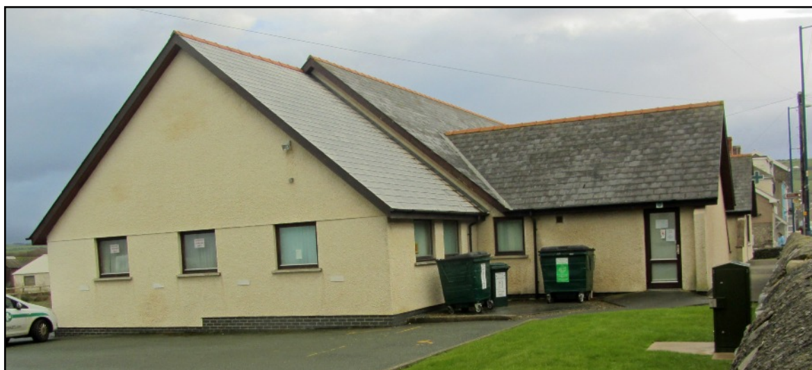
ABOVE The lower northern section of the building whose gable end faces the car park.
