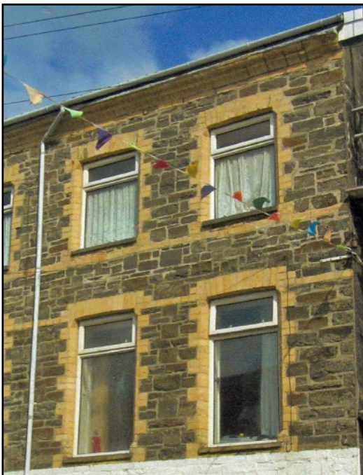
LEFT The front wall rubble stone has some large blocks and nicely squared and smoothed stones. This was more expensive. Shaped yellow bricks line the eaves like brackets supporting the overhang of the roof and yellow bricks are used to draw string courses linking all the front windows together. This photograph was taken in 2014. The windows are modern.
