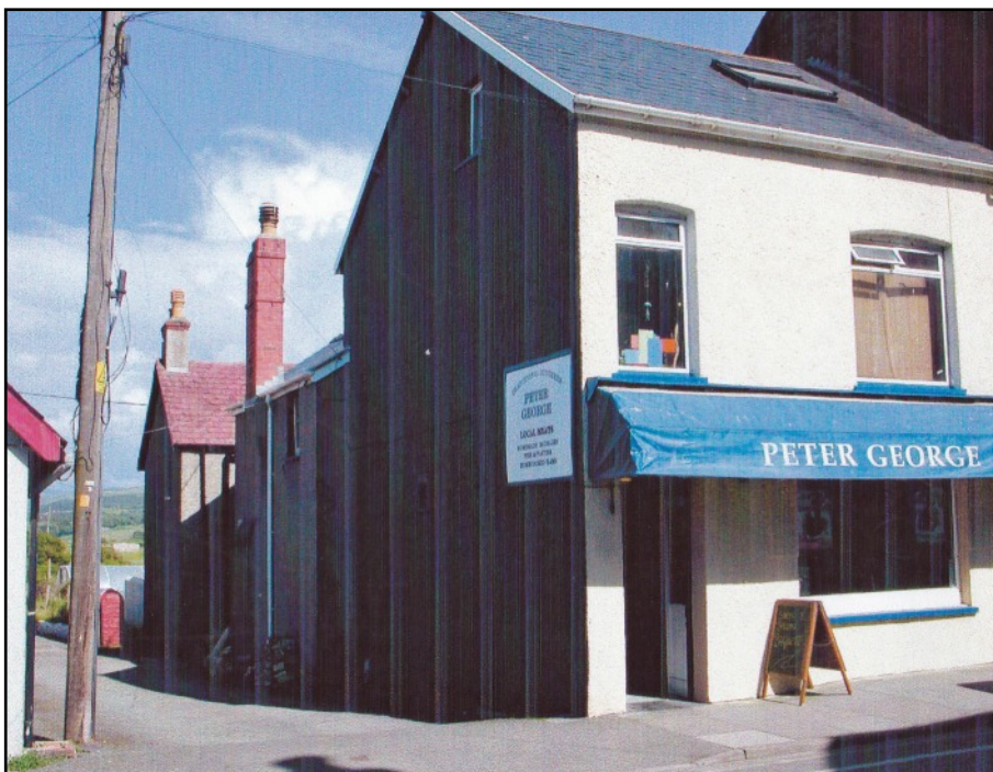
LEFT The side wall on the north which opens on to a lane is divided into five vertical sections. Almost joined to it is a barely two storey section with a roof at right angles to the main road which has a tall red brick chimney.
