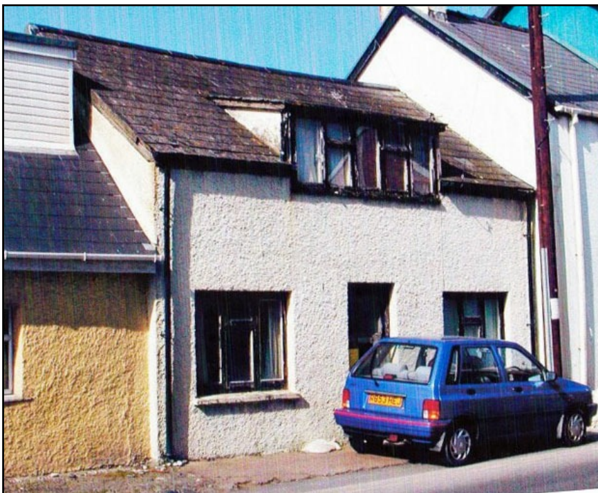
Leander in 2009. It had its dormer windows in the centre of the roof, under a nearly flat roof. The window frames were not the same, and the rendering on the wall was rough-cast.
