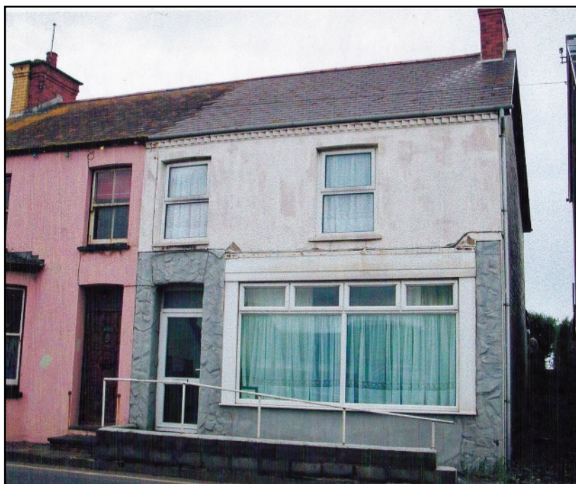
LEFT The house in April 2009 when it still had a shop front. Mock stone surrounded this and the front door, with smooth rendering below the shop window, and a board above for a shop name and perhaps a blind.
