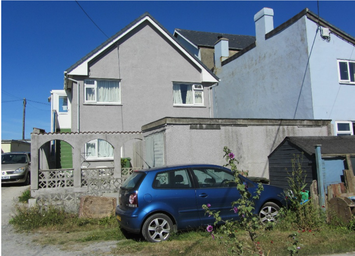
ABOVE This was the rear of the building in 2017. The entrance staircase to Kenlea is on the left which leads to a porch. There is a decorative patio area at the rear for that flat and there is a garage. The two bedrooms for Kenlea will have views across the railway, pasture and marsh to the hills beyond.
