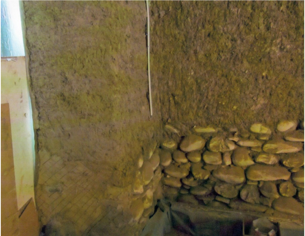
ABOVE Once the wall had turned the corner a doorway had been cut into it, and the width of the clom can be seen on the left.
