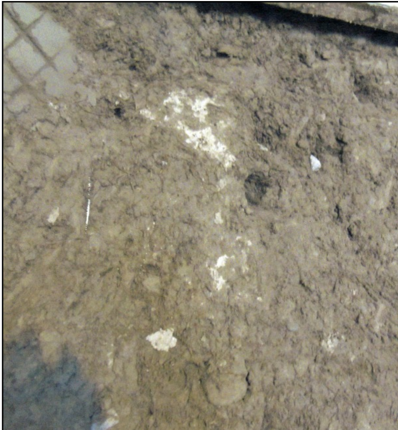
LEFT There were some holes in the mud - this was part of the rear wall. The white is remains of the plaster which had been stripped off but there were also small pieces of plaster embedded in the mud. The width of the mud wall can be seen in this photograph.
