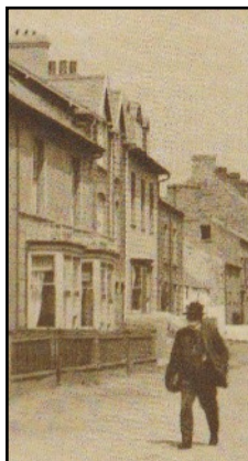
LEFT A detail from a postcard of the 1920s. Hafan is the fourth house from the left and had no dormer windows.
