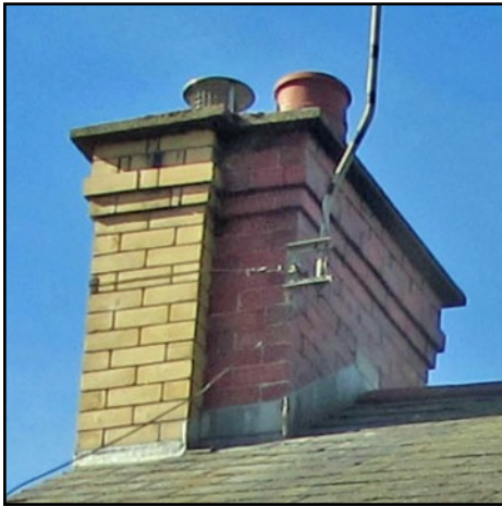
The chimney has two sections, one red brick, one yellow brick.
