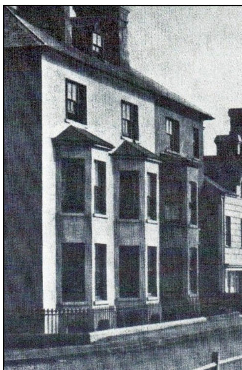
ABOVE This detail from a postcard shows the front of the hotel about 1906. There were sash windows, and a dormer window was added to the roof. There were two slab chimneys, Uppingham House next door had one as well. That houses were still separate and rendered a different colour. (Postcard Private Collection)
