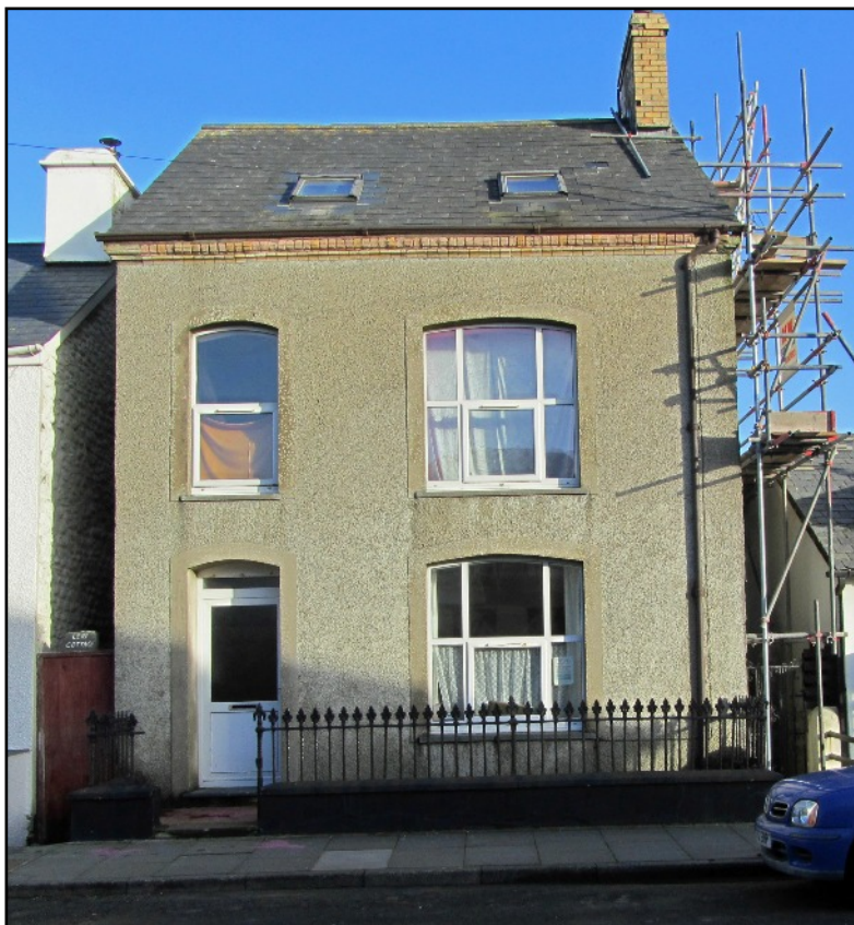
LEFT Gleaner when repairs were happening to the slate hung side.
