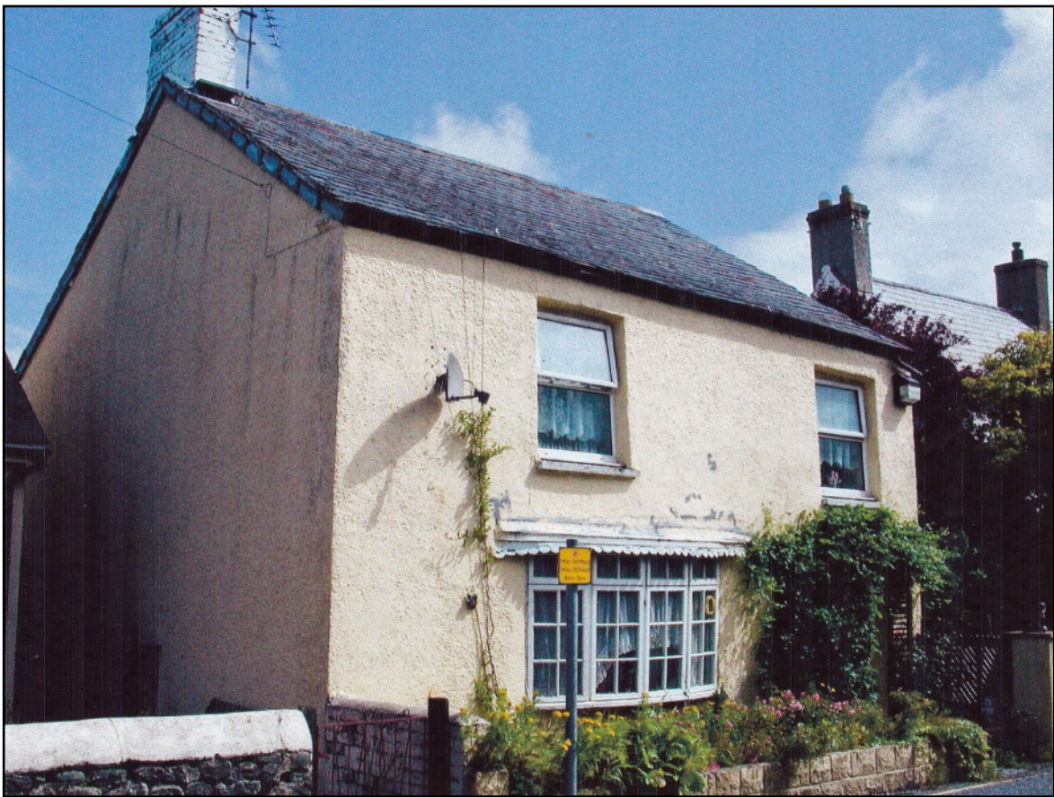
ABOVE The house in 2009 had lost its easternmost chimney and had a canted oriel bay window decorated at the top by a strip edged with small curves. A trellis porch over the front door was covered with creeper. The upper windows, as today were modern, larger and squarer than the old windows, but in the pattern of a sash window. The chimney was whitewashed brick. There was a trellis wall with panels enclosing the east end of the garden. The front door is on the east side of the front.
