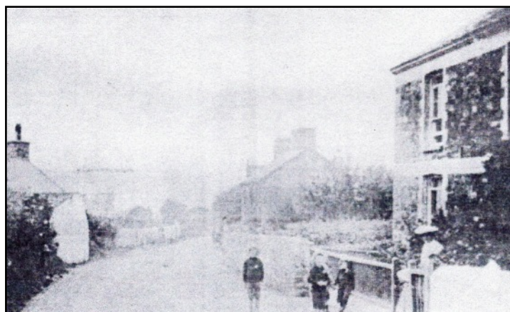
ABOVE Glasfryn House in the time of the Herbert family. The house was exposed rubble stone, its windows edged by pale coloured bricks, and with two broad bands of plaster, not common in Morfa Borth. There were sash windows, and they were open as it was summertime. There is a lady (Mrs Herbert?) with a little girl at the gate. The wall round the narrow front garden was topped by railings, and there were plants climbing up part of the front wall of the house (Y Tincer, 1998, Aberystwyth Public Library).
