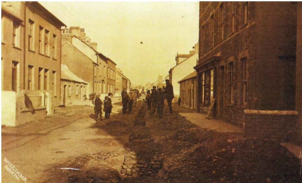
There is a glimpse of Glasfryn on this old postcard, the photograph taken when a trench was being dug in the road. Glasfryn is the sixth from the left, easy to see from its overhanging roof. It had some substantial chimneys. The walls were rendered, the side wall in a pale colour. The windows were smaller and the ground floor did not have a bay window. On the right is the tall London House with its shop. (Postcard courtesy of the Amgueddfa Ceredigion Museum).
