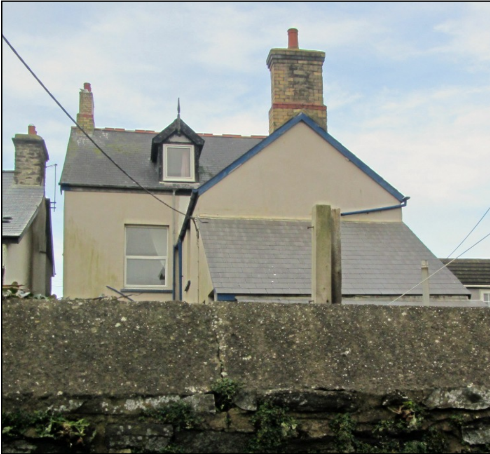
ABOVE Glan Dylan from the small lane at the rear of its garden. The house has a substantial two storey wing which was already there on the 1904 map. It has a Victorian coloured brick chimney - suggesting this was where the original kitchen had been. There is also with a lean-to extension on the end of the wing. The windows are modern.
