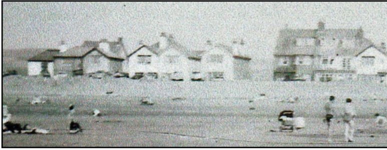
LEFT The gap into which Ger-y-môr would be built. To the left are the three houses, ending with Kingswood, and beyond and set back was a house called Panteg joined on to a 'Canteen Stores' which became a 'Spar' on the site of
