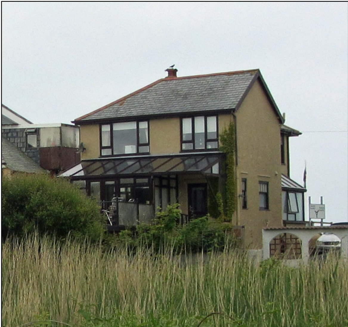
The rear of the house from the footpath. It has a glazed verandah roof protecting the back door, and a sun room extension built below it. Windows on the top floor would give a view across Borth's common land to the hills.
