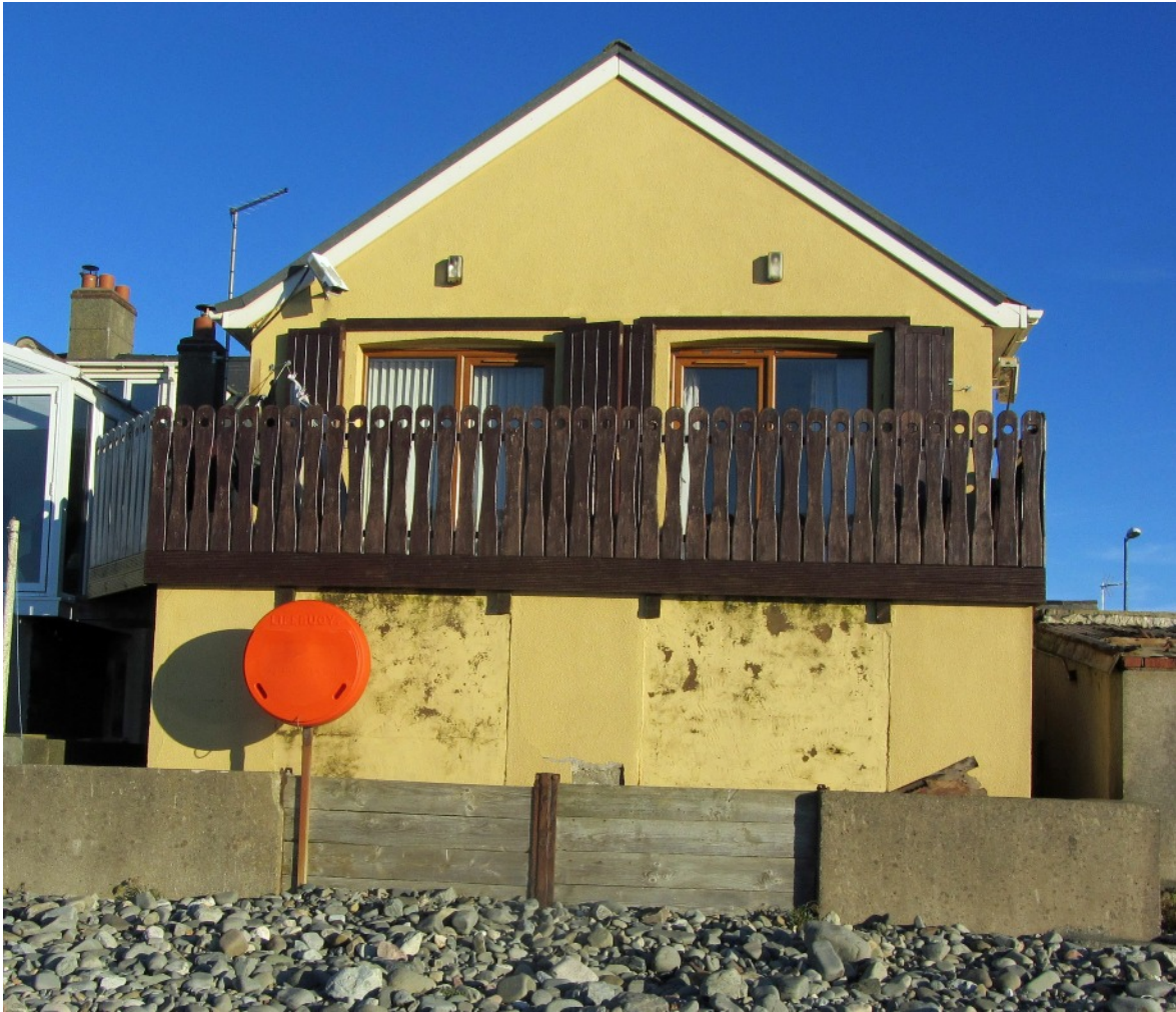
The beach side of the house in 2016. Shutters protect the windows and below the balcony panels protect the building from the sea during bad storms.
