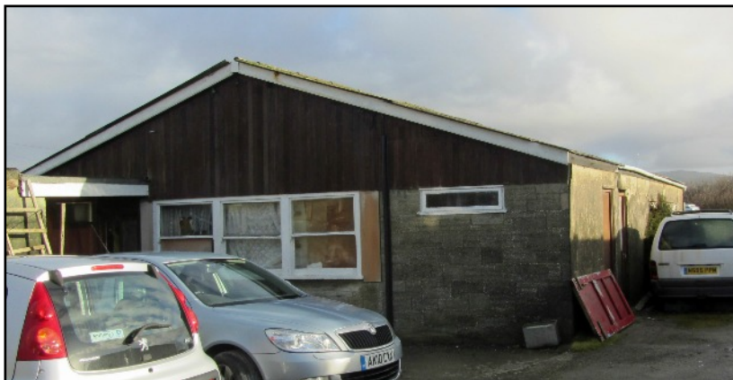
LEFT The large building at the rear in 2018.
